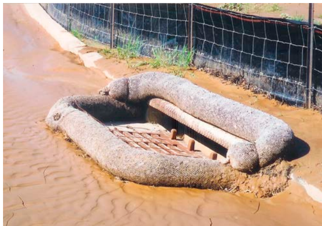
Figure 4 Compost filter sock curb inlet
