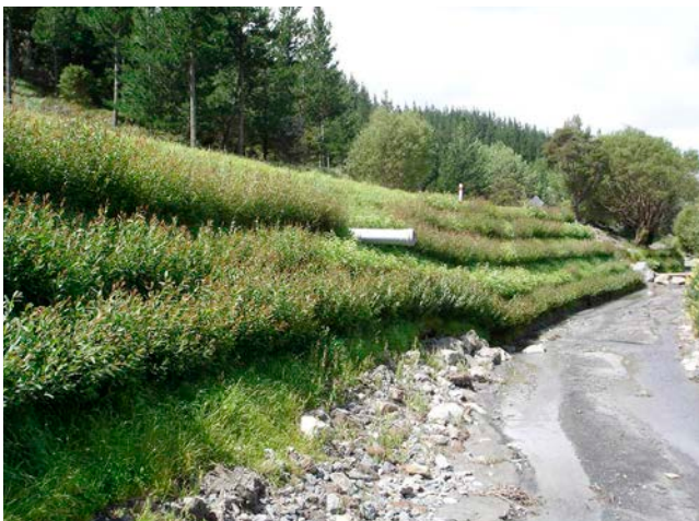
Figure 6 Vegetated compost filter socks
