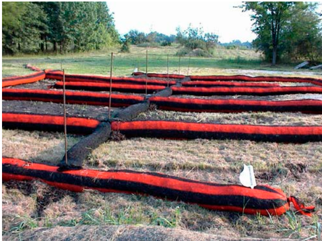
Figure 5 Compost filter sock biofiltration system
