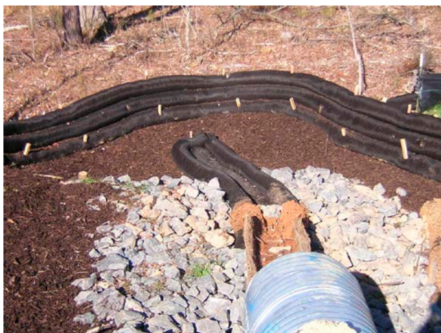
Figure 2 Compost filter socks used for capturing sediment
