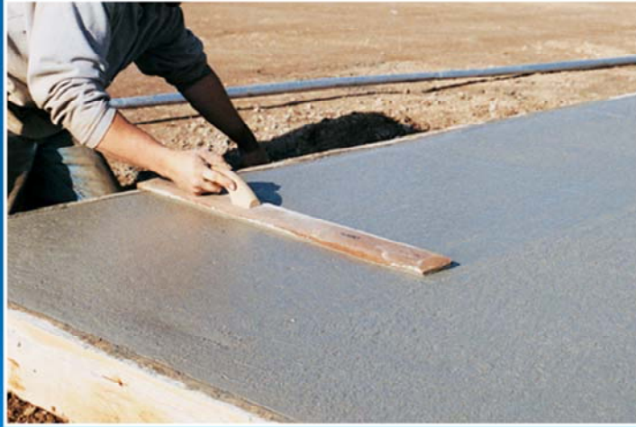
Finishing Flatwork (v.0515)
