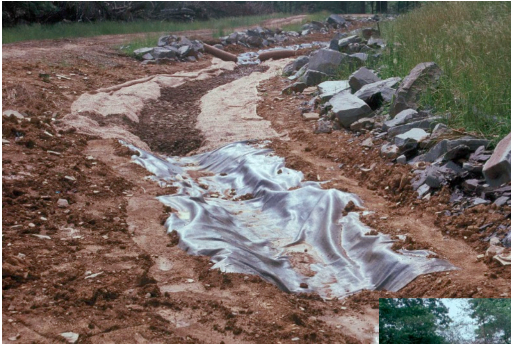
Restoration of stream channel following mining
