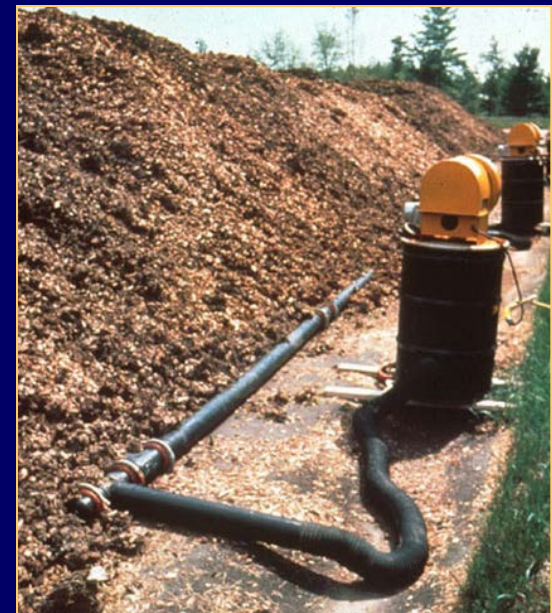
Forced aeration, Idaho
