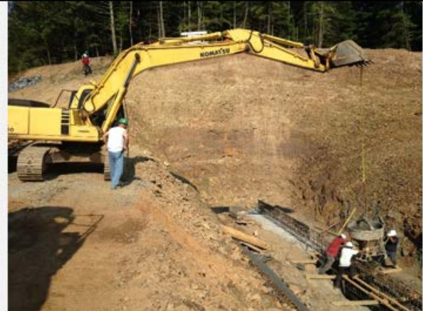
Photo 8 Excavator and bucket utilized to convey concrete
