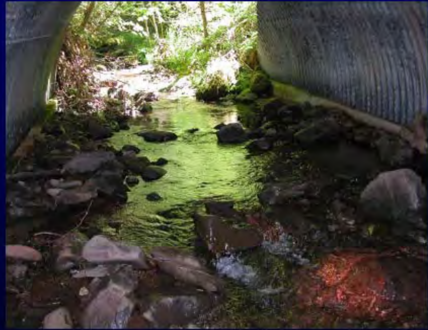
Stream simulation 21 years after construction
