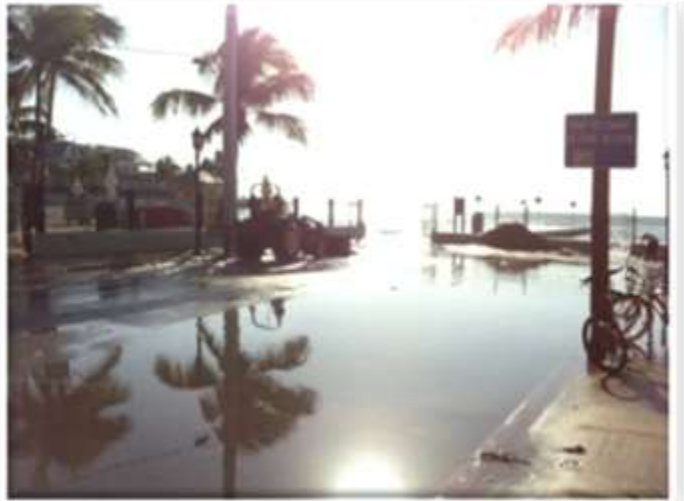
Duval Street high tide flooding
