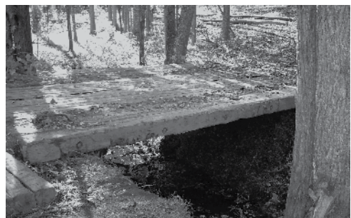
Portable timber bridge
