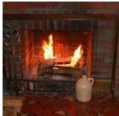
Fireplace 10% efficient $59 per million Btu's
