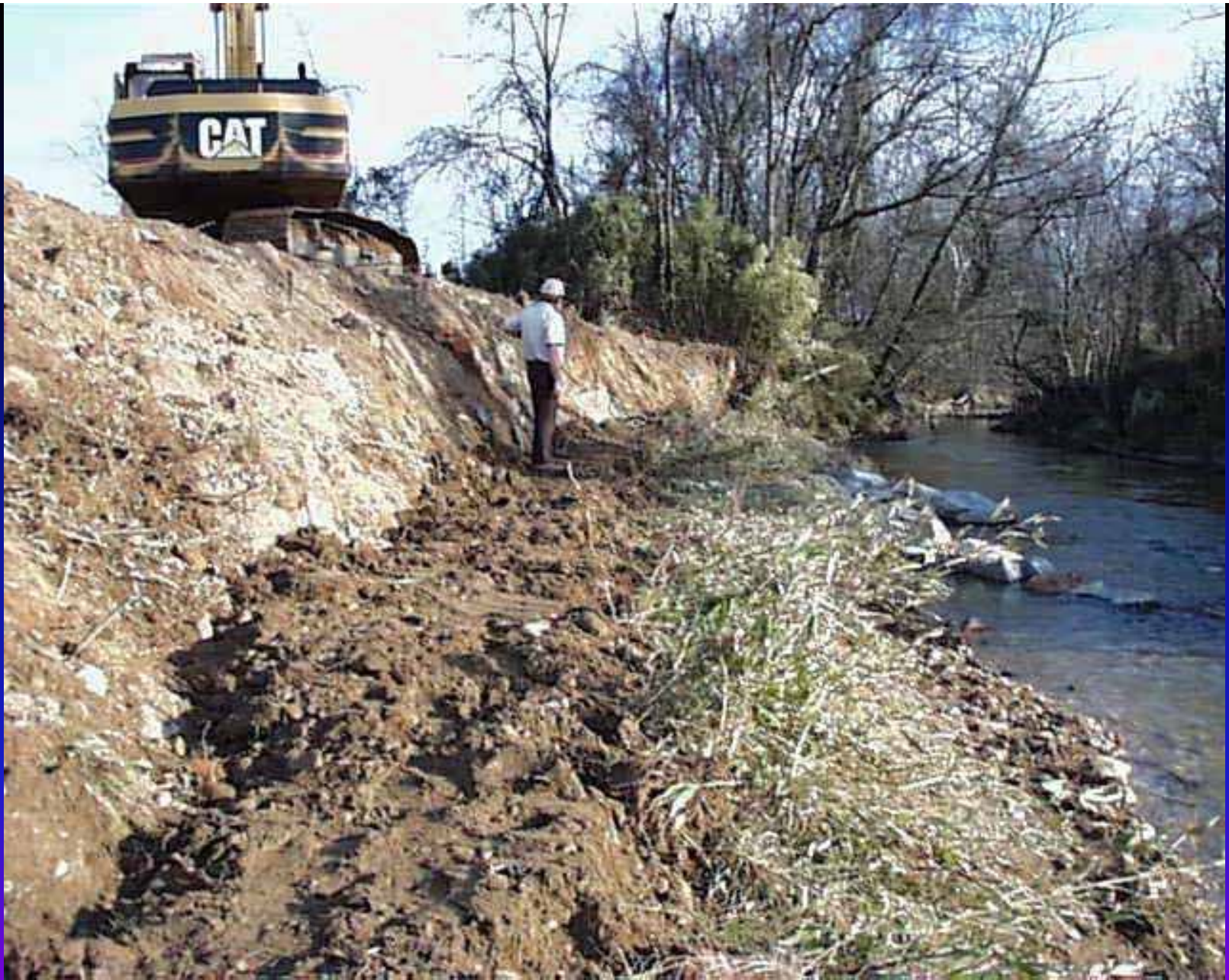
Brush Layering with Rock Vanes
