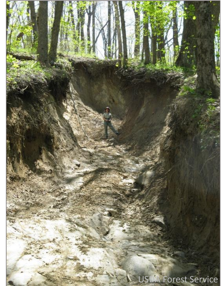
Gully erosion, Mississippi
