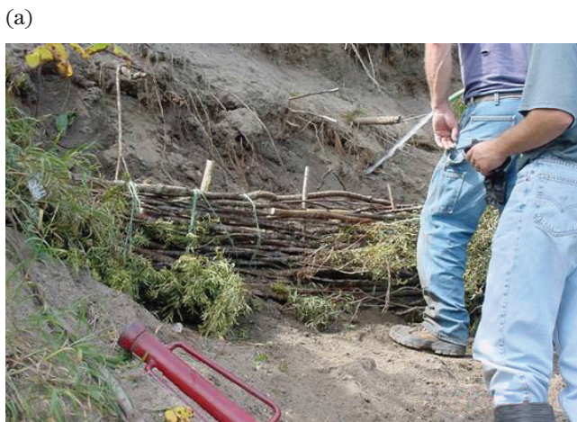
Figure TS14I-34 (a) Wattle fence immediately after construction; (b) 1 year later
