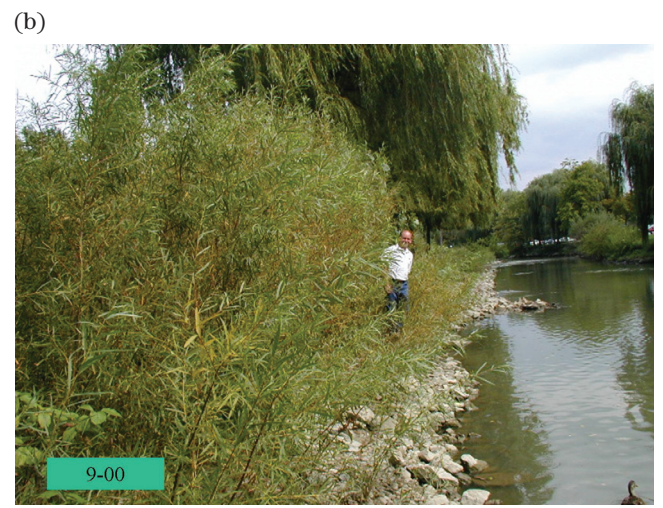
Figure TS14I-28 (a) Brush mattress being installed; (b) Brush mattress after one growing season
