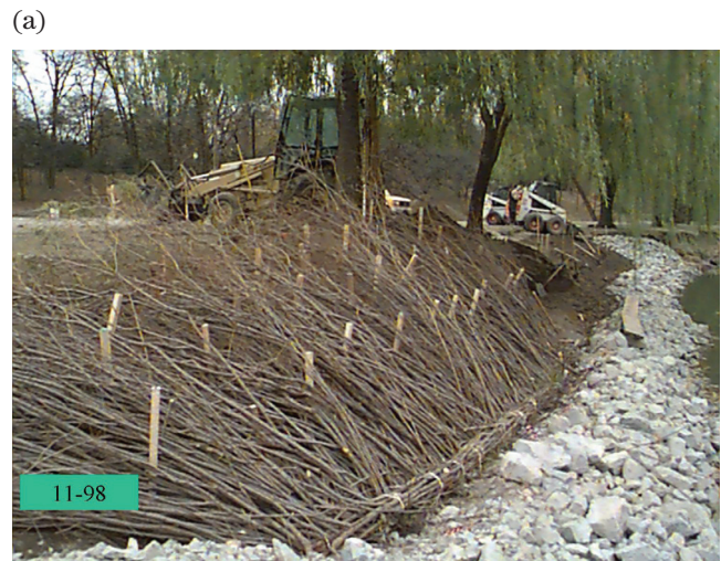
Figure TS14I-28 (a) Brush mattress being installed; (b) Brush mattress after one growing season
