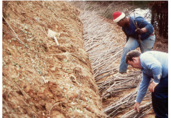
Figure TS14I-26 (a) Excavation of the brush layer bench; (b) Cutting placement ( Photo courtesy of Robbin B. Sotir & Associates, Inc. )
