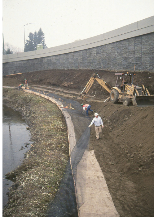
Figure TS14I-31 Geogrid wrapping of soil lift ( Photo courtesy of Robbin B. Sotir & Associates, Inc. )
