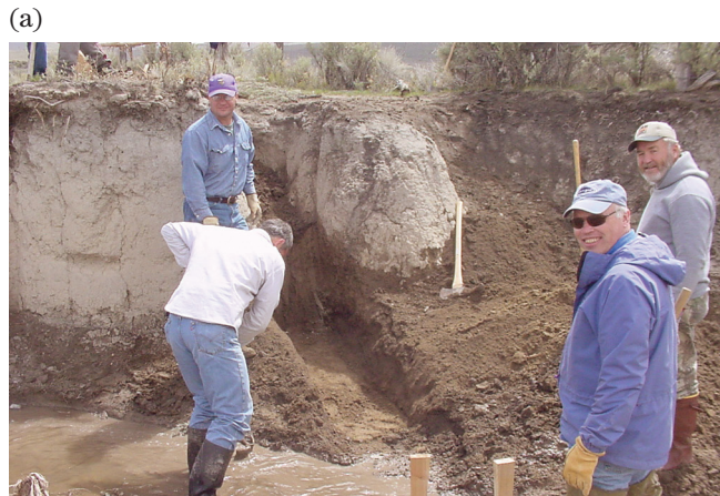
Figure TS14I-13 Brush spur being installed
