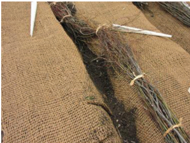
Figure TS14I-40 Combining fascines and fabric
