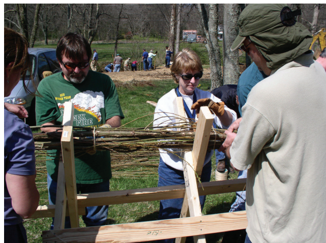
Figure TS14I-18 Assembling fascines
