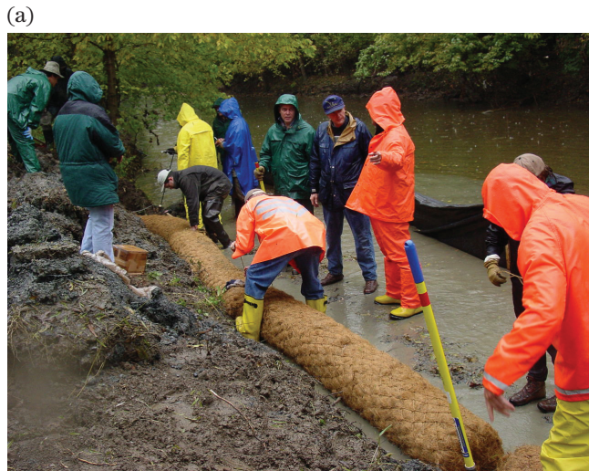
Figure TS14I-8 Installation of coir fascines: (a) Anchoring; (b) Tying of the coir fascines together ( Photos courtesy of Robin B. Sotir & Associates, Inc. )
