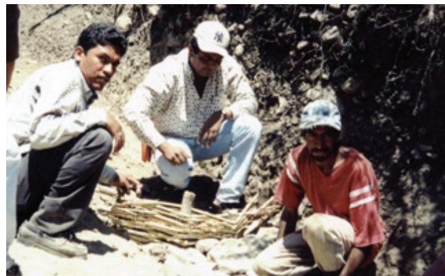
Figure TS14I-36 Brush wattle fence to deter erosion in a gully
