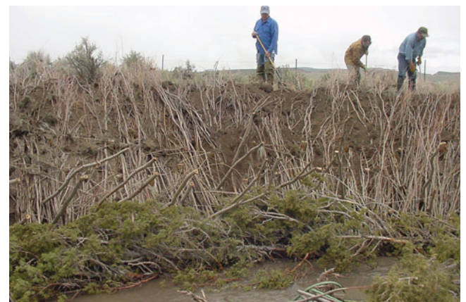
Figure TS14I-10 Brush/tree revetment over poles and a brush mattress
