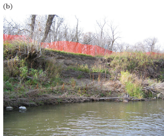
Figure TS14I-34 (a) Wattle fence immediately after construction; (b) 1 year later
