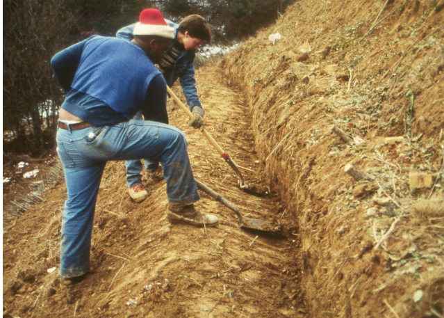
Figure TS14I-26 (a) Excavation of the brush layer bench; (b) Cutting placement ( Photo courtesy of Robbin B. Sotir & Associates, Inc. )
