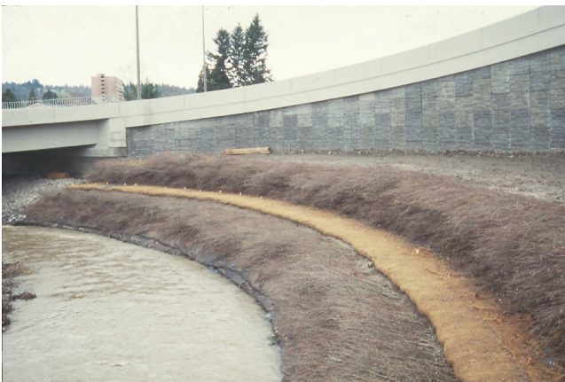
Figure TS14I-32 Completed VRSS ( Photo courtesy of Robbin B. Sotir & Associates, Inc. )
