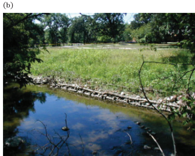
Figure TS14I-17 (a) Live cribwall under construction; (b) After first growing season
