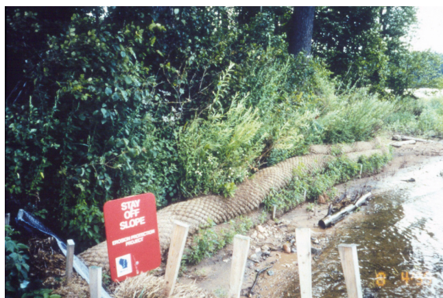
Figure TS14I-9 Stacked coir fascines using woody vegetation ( Photo courtesy of Hollis Allen )
