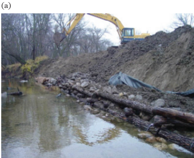
Figure TS14I-17 (a) Live cribwall under construction; (b) After first growing season
