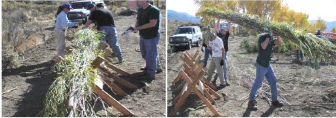
Figure 18-9: Fabrication of a Live Fascine Bundle
