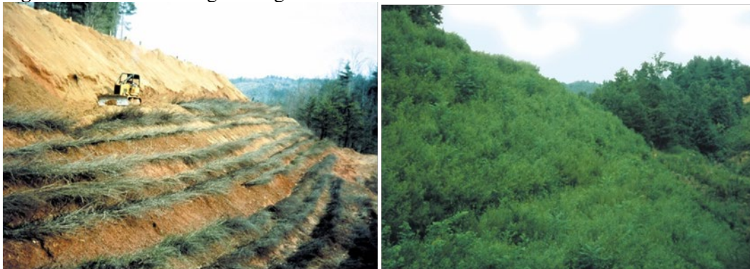
Figure 18-2: Soil Bioengineering Provides Soil Reinforcement and Reduces Surface Erosion
