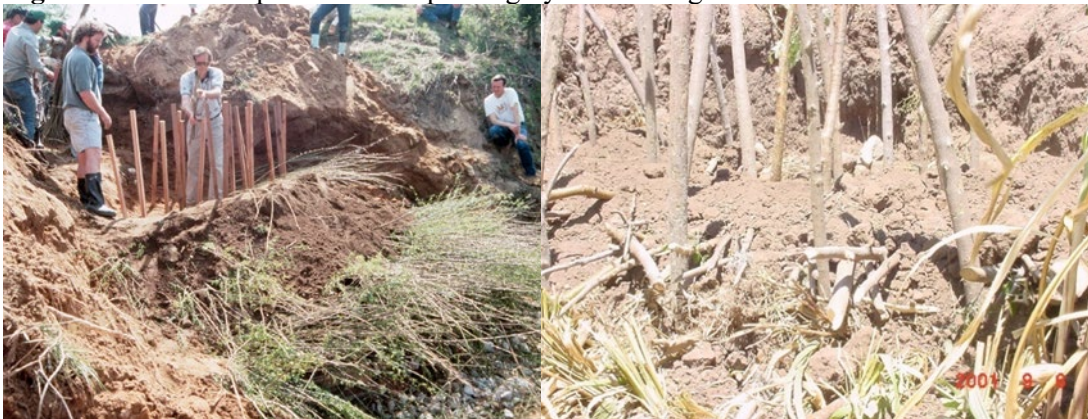
Figure 18-15: Examples of Branchpacking Systems Being Installed
