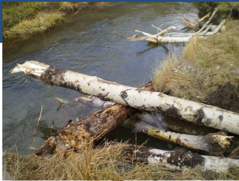
Live clumps and flexible wood for toe protection
