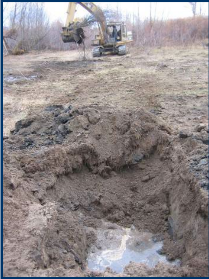
Excavate hole to water table
