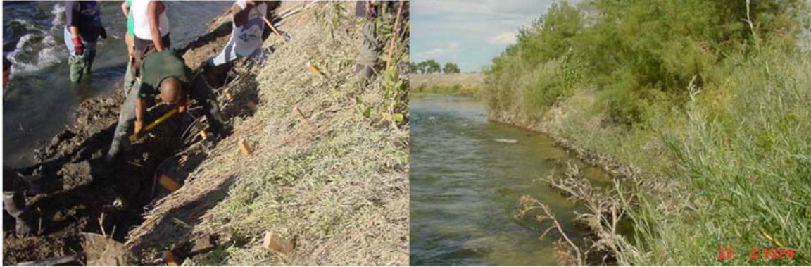
Figure 4: Brush Mattress under construction and after 2 years.
