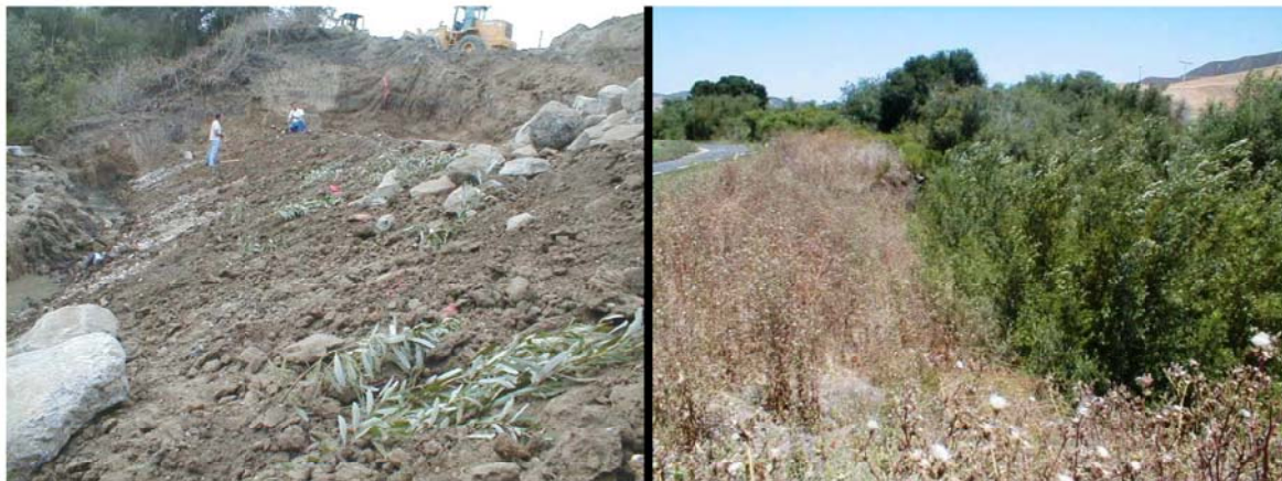
Figure 1: Vertical bundles placed behind a stone toe. Under construction and after 4 years
