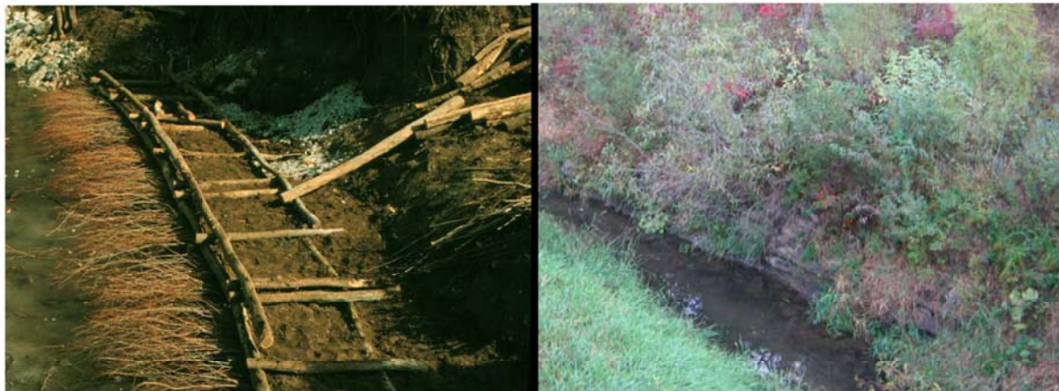
Figure 2: Log Crib. Under construction and after 10 years
