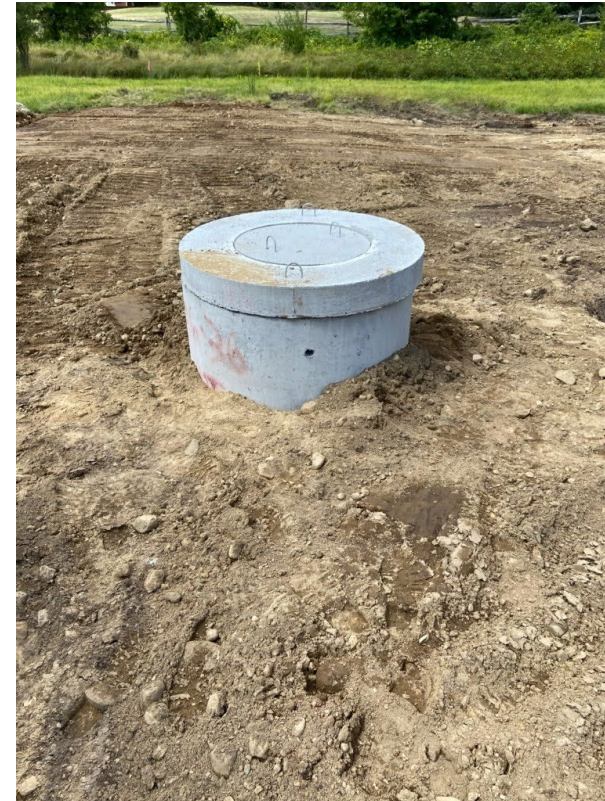
Typical concrete tile excavated well
