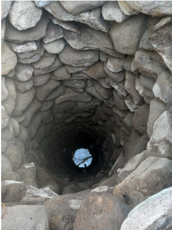
Vintage stone lined hand-dug well
