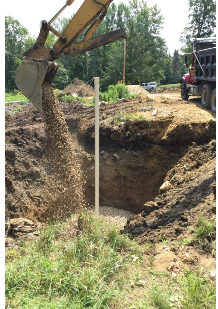
Filling in around the casing
