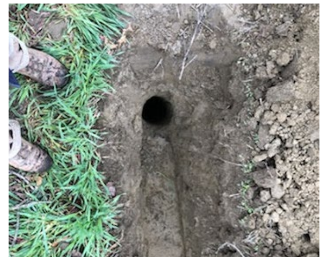
Point wells are often augered by hand and sleeved and pounded in the ground.
