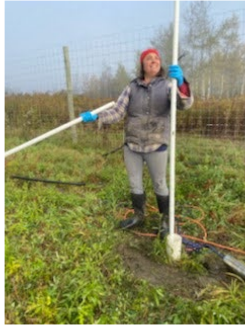
Add pipe and lower the well developer into the casing
