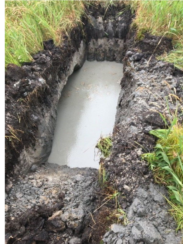
Test pit after 3 hours
