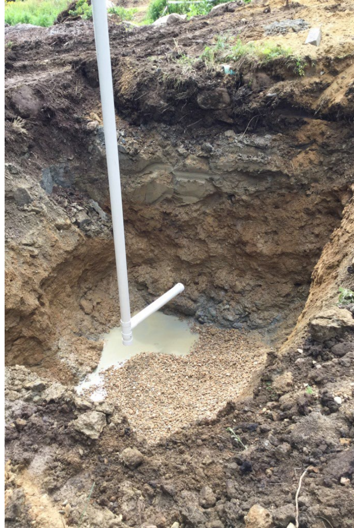
Setting the casing
