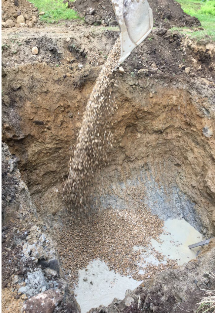
Preparing the base
