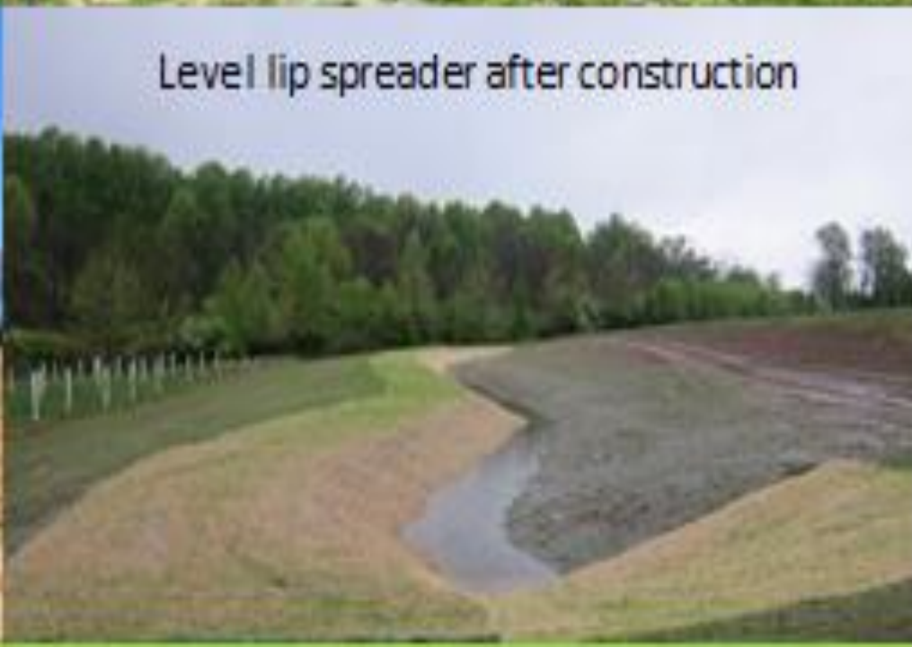
Level-lip spreader during construction
