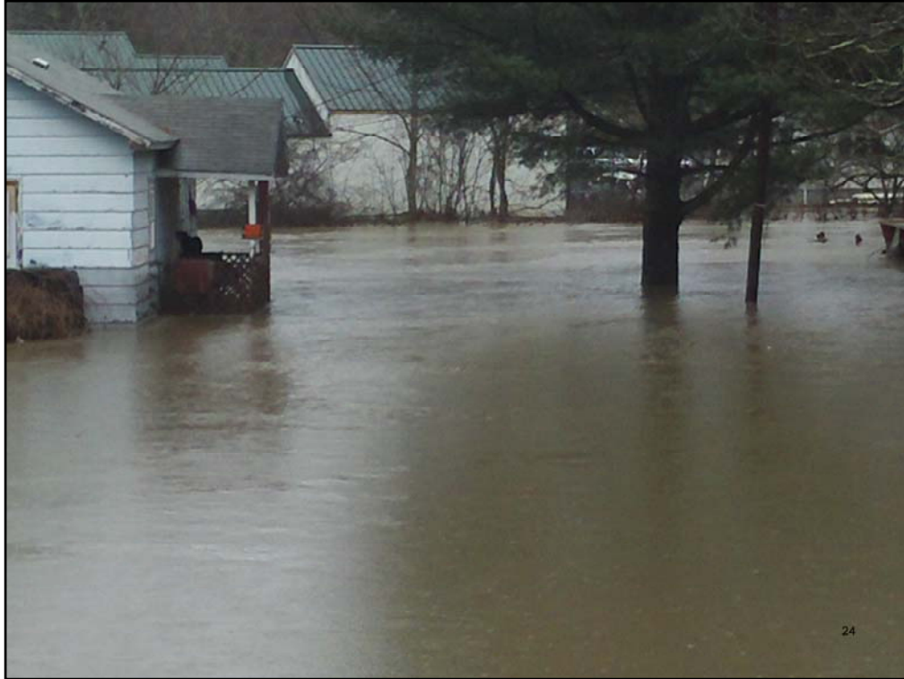
Another example of flooding in the watershed. See the high water mark on the house siding, just below the window.
