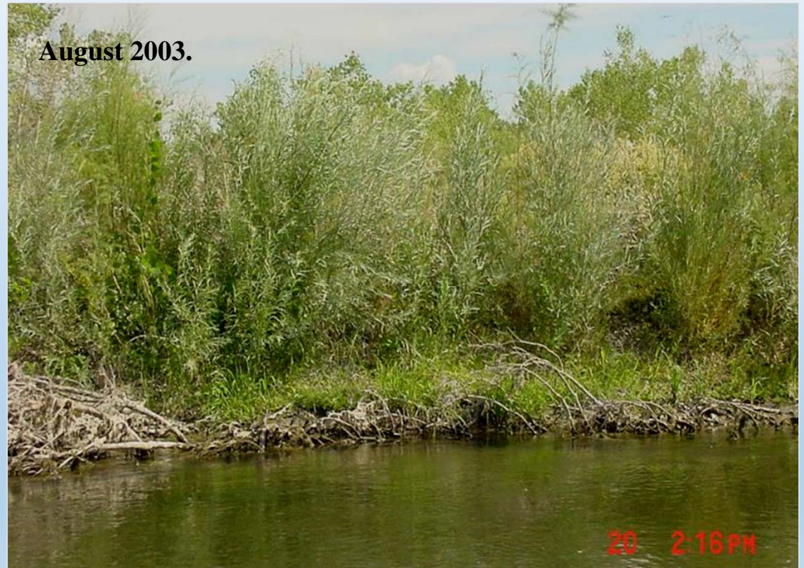
Vertical bundle and brush (juniper) revetment
