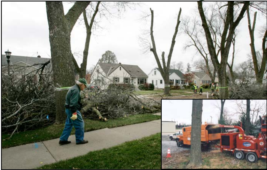
Tree removal and sanitation
