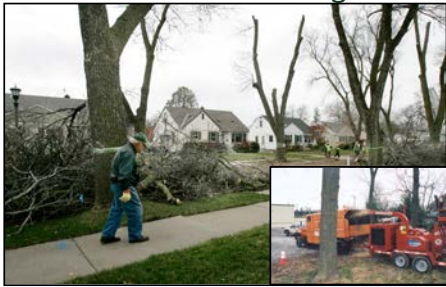
Tree removal and sanitation
