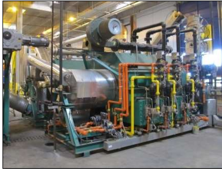
The Tucker RNG biomass gasification system developed in partnership with USFS.
